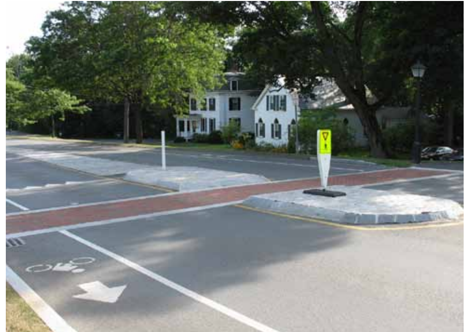
Improved crossing treatment with median island in Amherst, Massachusetts.
