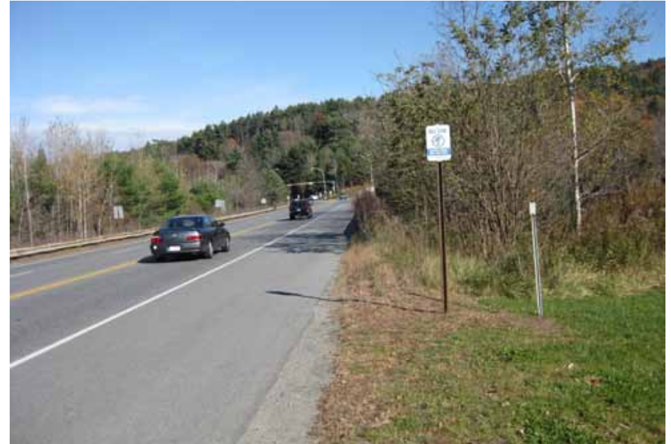
Pedestrian crossings at Buck Road/Hanover Town Garage on route 120 are a concern.
